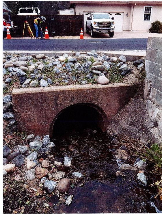
Figure 8: Existing Inlet Structure with 42-inch Pipe
