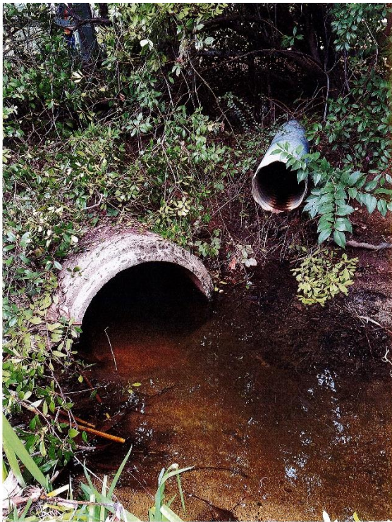
Figure 7: Existing Outlet Structure
